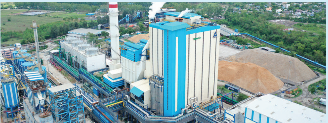
New High Pressure Recovery Boiler at the ITC Paperboards & Specialty Papers Manufacturing unit, Bhadrachalam, Telangana
