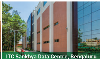
ITC Sankhya Data Centre, Bengaluru
